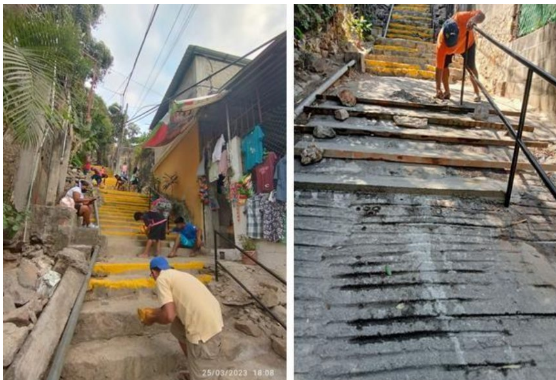
Photo 15. Follow-up of Stair Painting and Ramp Restoration. Source: Ramirez, 2023.
