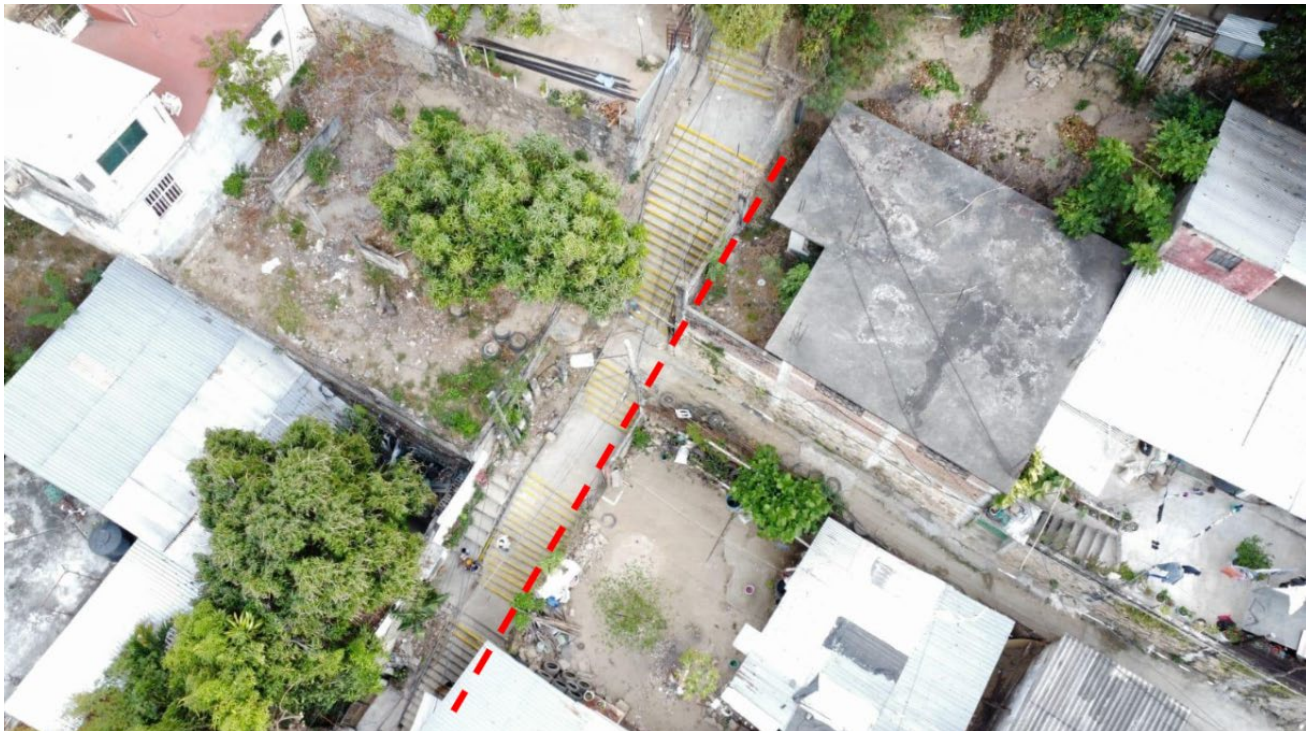
Photo 19. Slope on the Abasolo Walkway.
