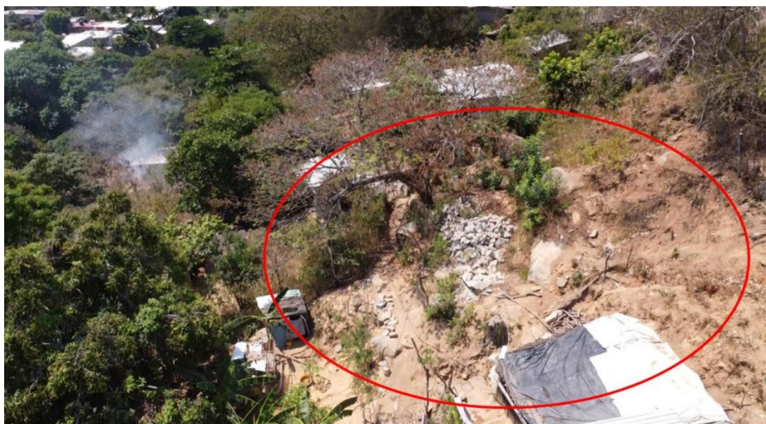
Photo 21. Risk due to a Landslip.
