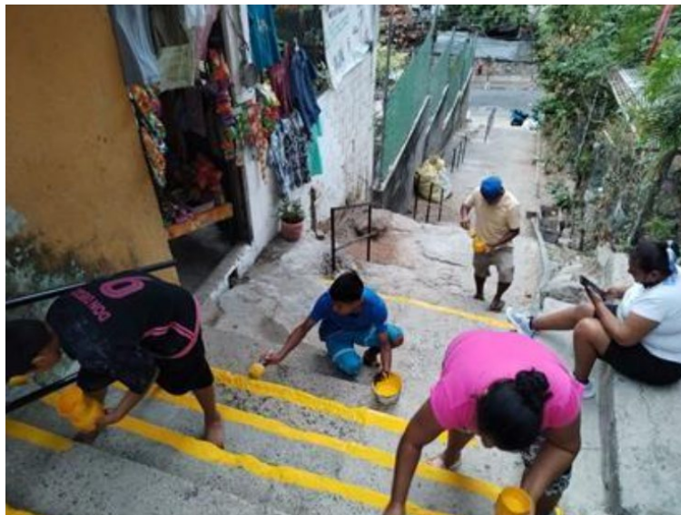
Photo 16. Rehabilitation of Abasolo Walkway. Source: Ramirez, 2023.
