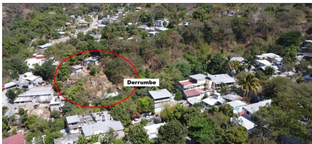
Photo 22. Risk due to a Landslide.
