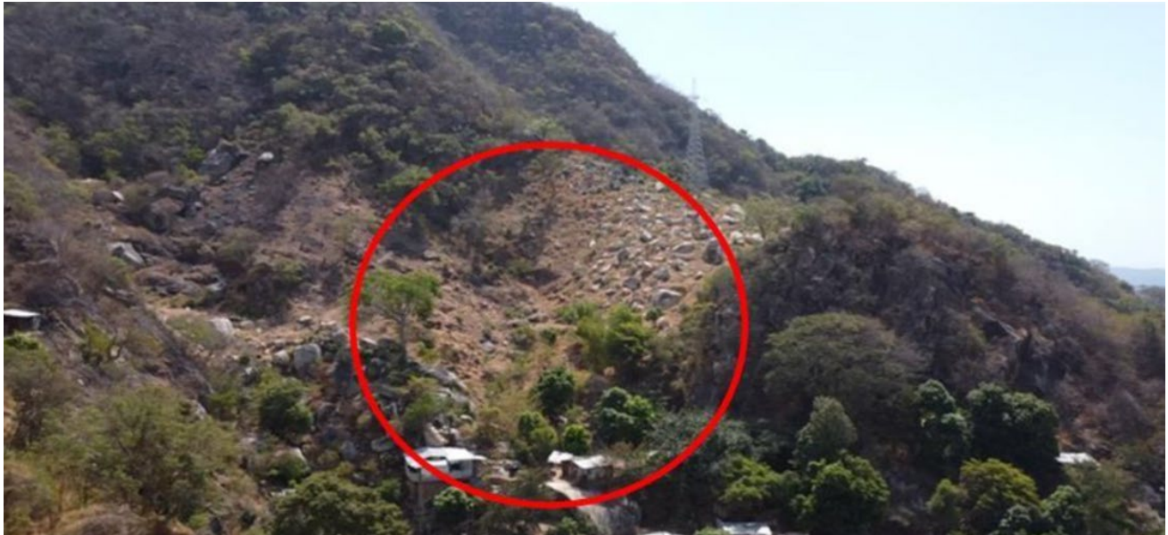
Photo 23. Risk due to Falling Blocks
