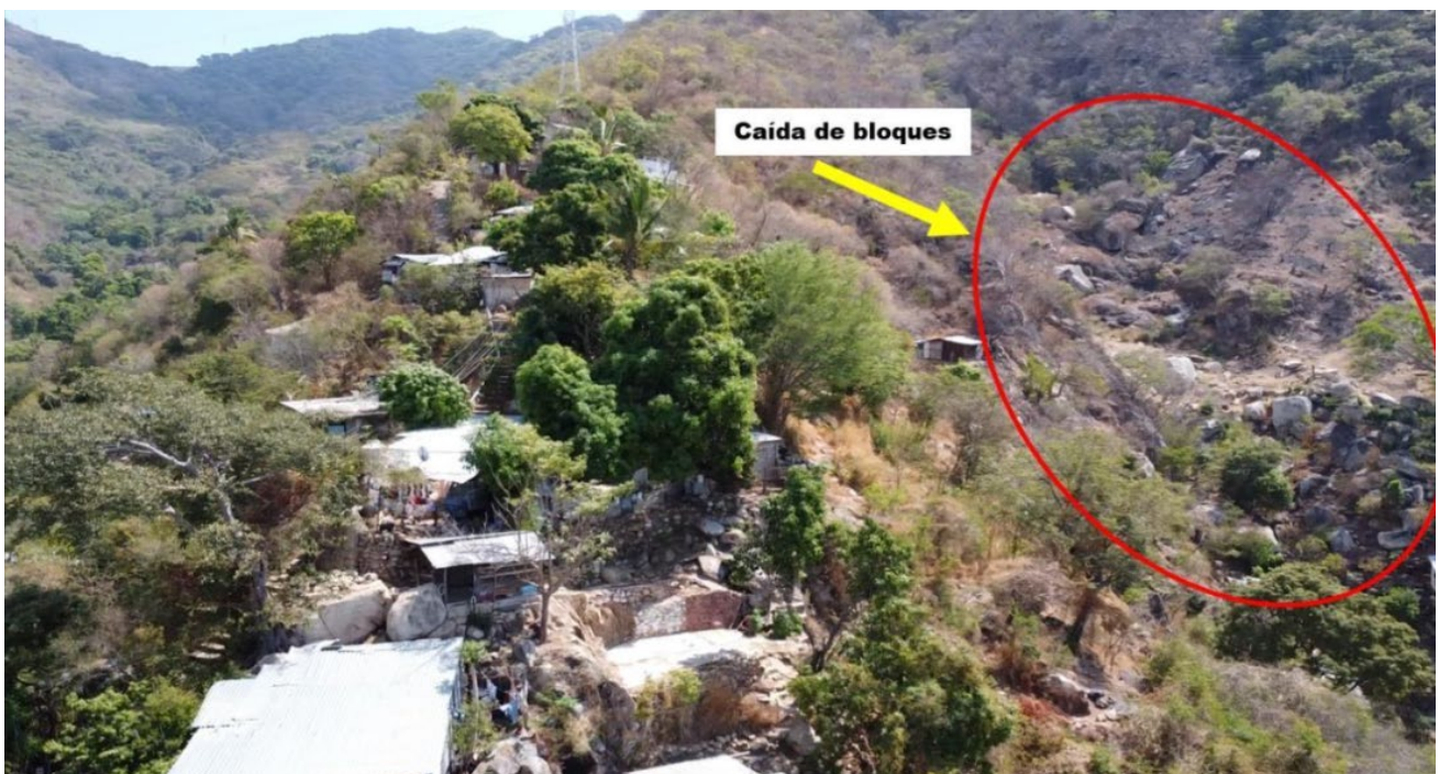
Photo 24. Risk of Blocks Falling on Houses.
